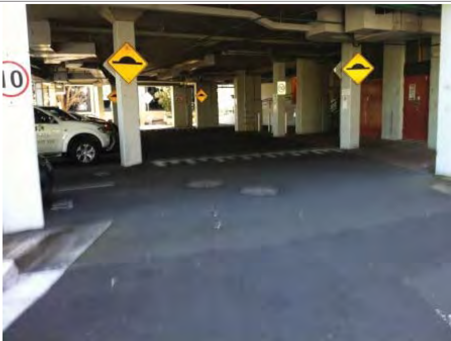
Photo 5.1.1.2 – Undercroft vehicle parking beneath council administration building, looking towards the north
