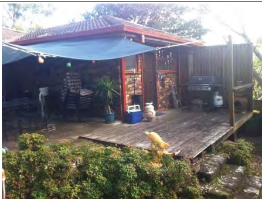
Photo 0.2 – View of north eastern side of residential dwelling
