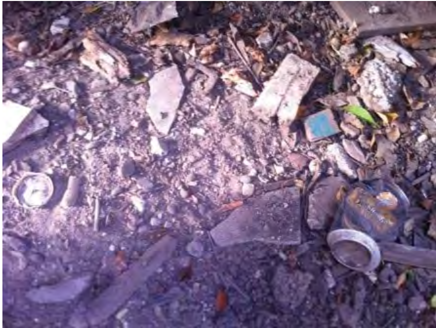
Photo 5.6.1 – Fragments of fibrous cement sheeting beneath residential dwelling in Lot C in DP386283.
