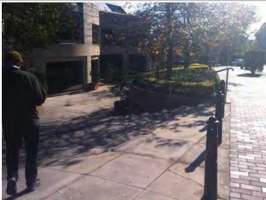
Photo 5.1.2.2 – View of eastern side of building
