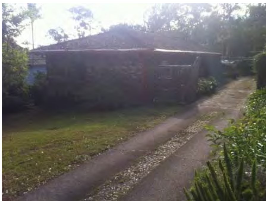
Photo 0.1 – Southern view of residential building
