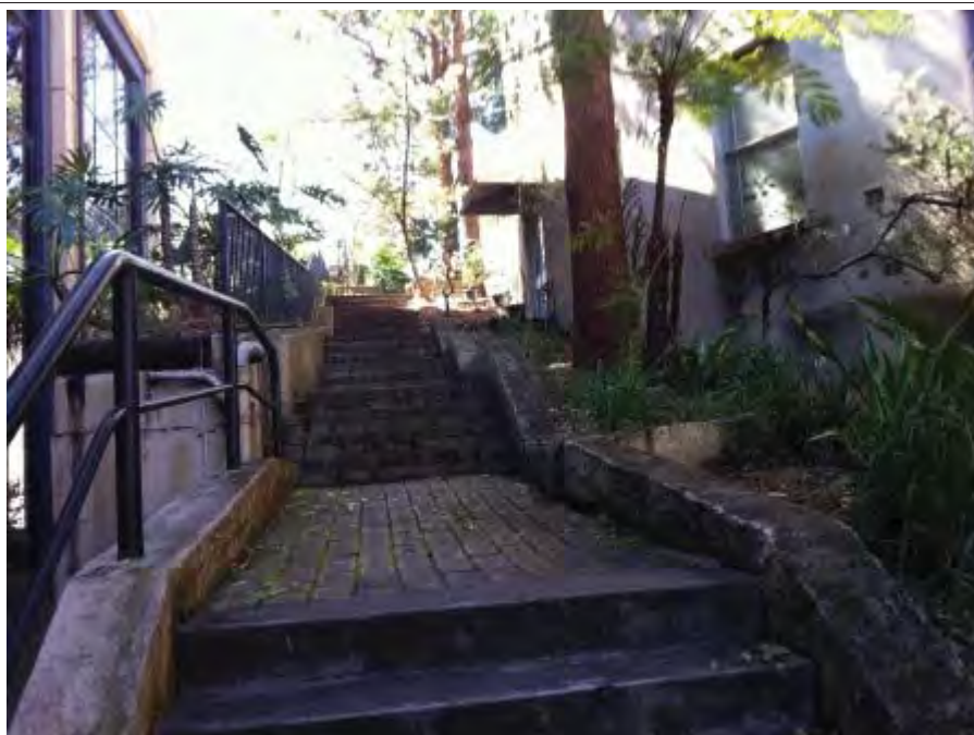
Photo 5.1.1.9 – Paved stairs and gardens along northern boundary of the site, looking towards the east
