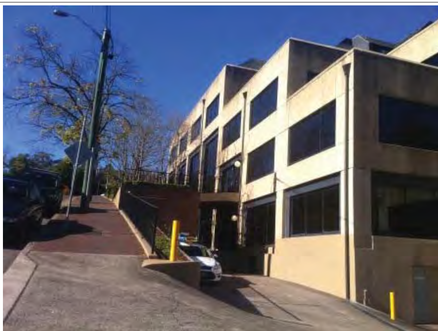
Photo 5.1.2.3 – View of northern side of building
