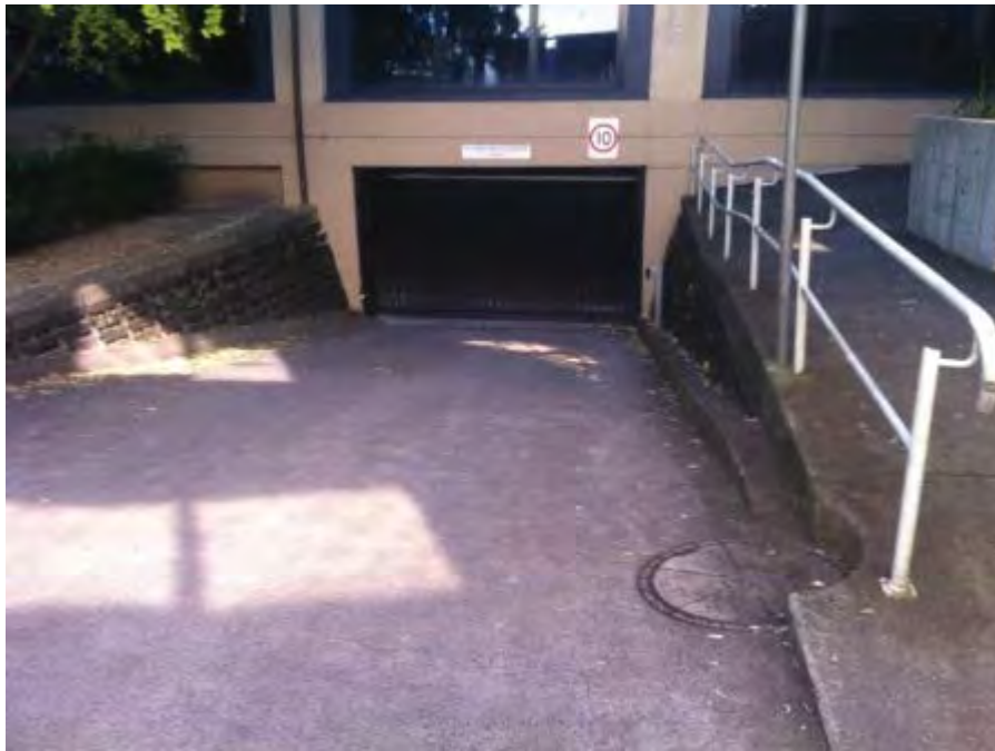
Photo 5.1.2.6 – View of entry/exit basement driveway on southern side of building
