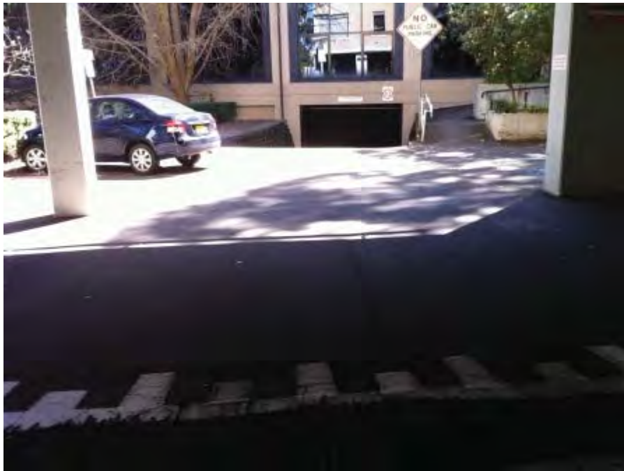
Photo 5.1.1.3 – Undercroft vehicle parking beneath council administration building, looking towards the north
