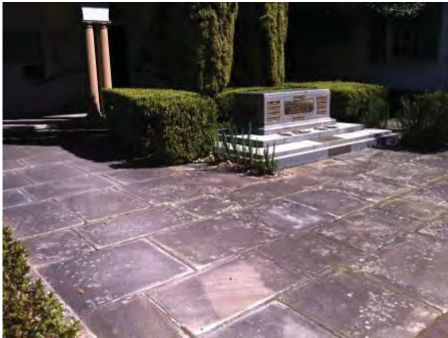
Photo 5.1.1.1 – Paved area on eastern side of council chambers building
