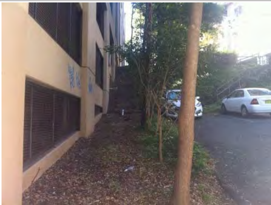
Photo 5.1.2.7 – View of south western side of building
