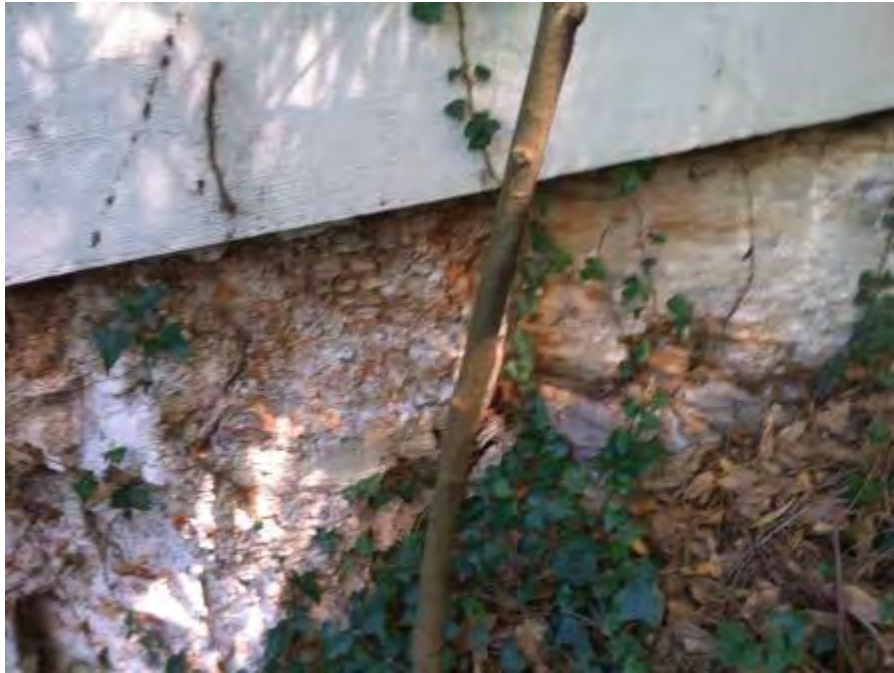
Photo 5.4.1 – Exposed natural clayey shale observed beneath the building slab on the southern side of the council administration building
