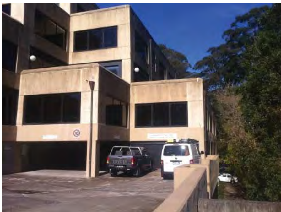
Photo 5.1.2.4 – View of western side of building
