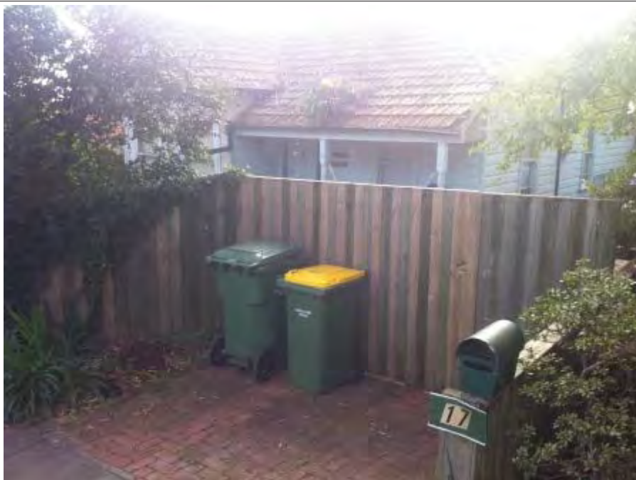
Photo 5.1.4.1 – View of southern side of building
