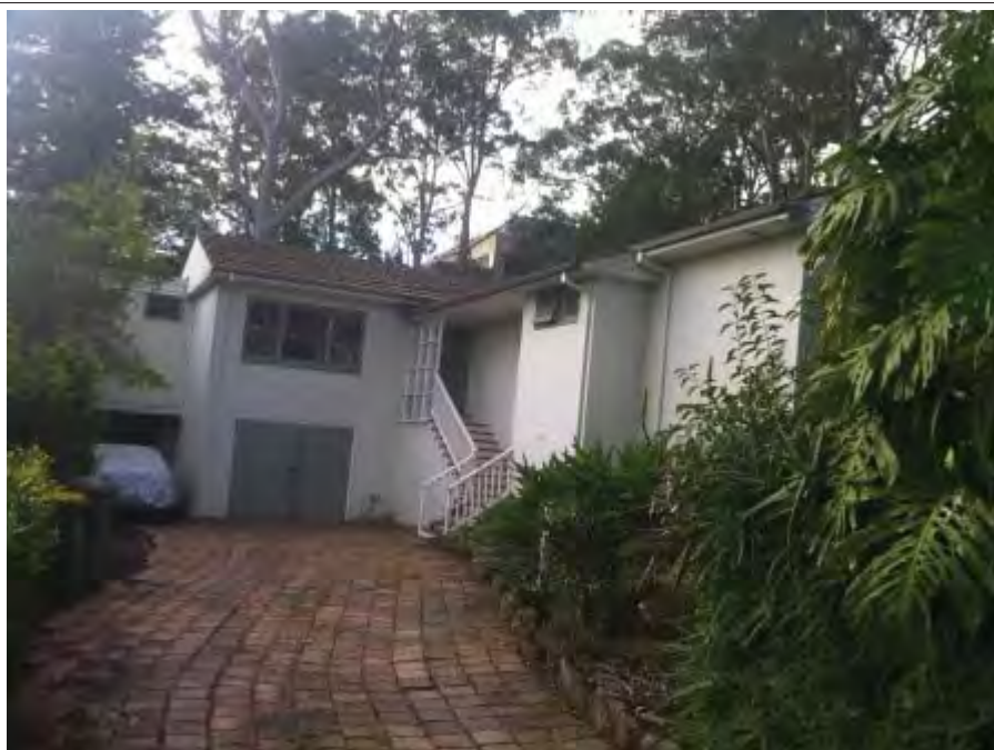
Photo 5.1.3.1 – Southern side of residential building
